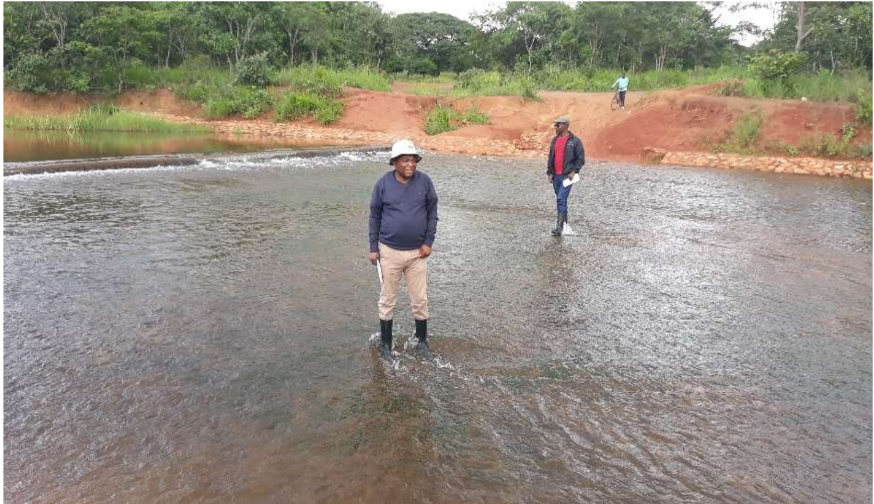
Figure 7: Concrete lined spillway still intact
