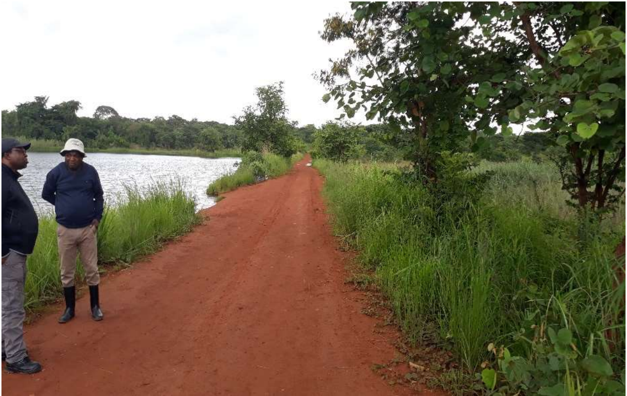
Figure 6: Embankment overgrown with grass and shrubs
