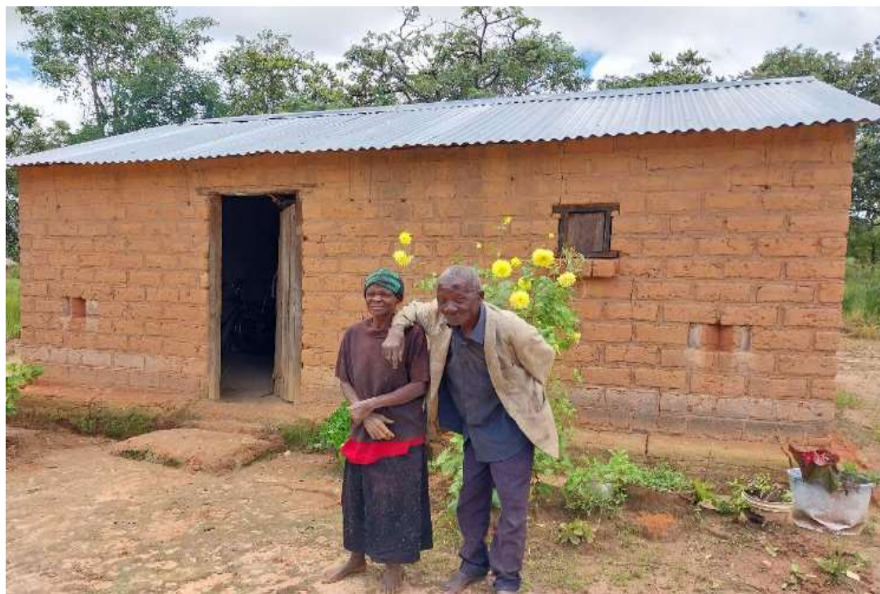
Figure 23: Brick House for Mr. Peter in the farm Block
